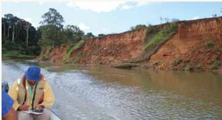
Erosion along the river banks
